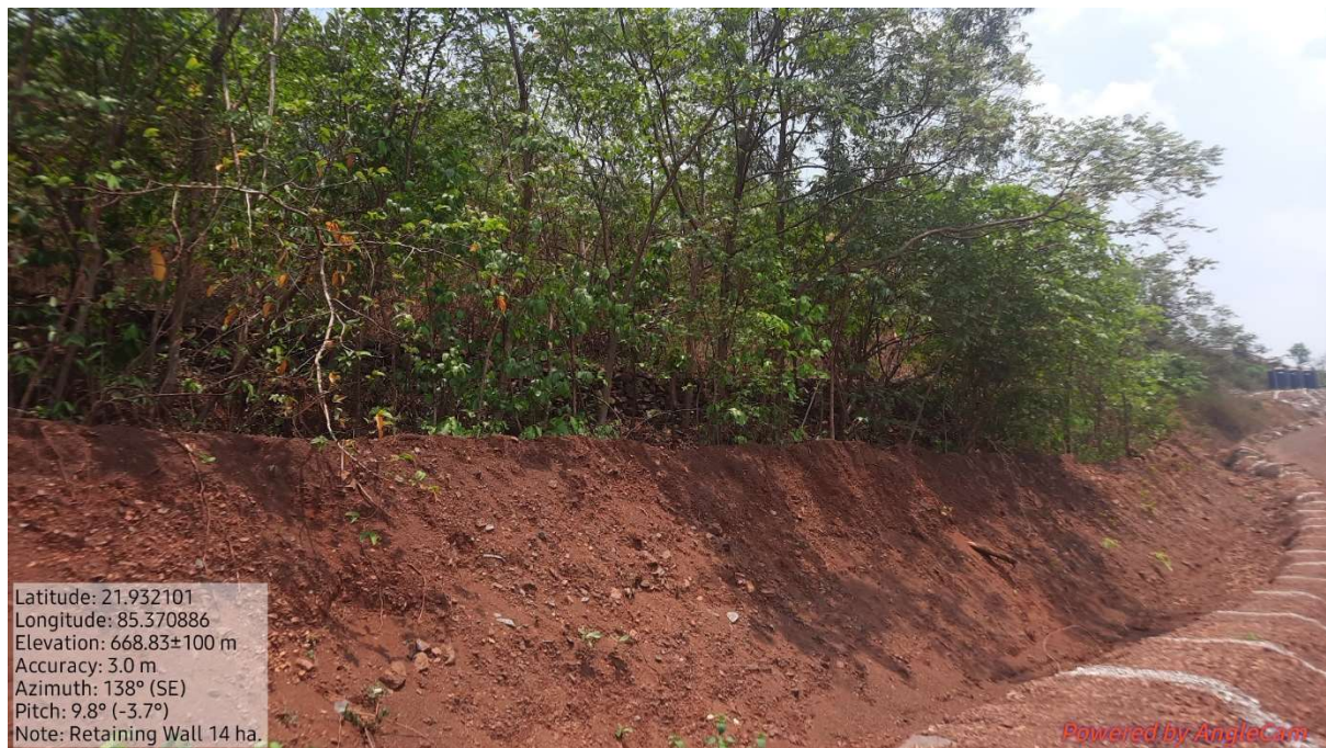
PHOTOGRAPH: 3 PHOTOGRAPH SHOWING RETAINING WALL
