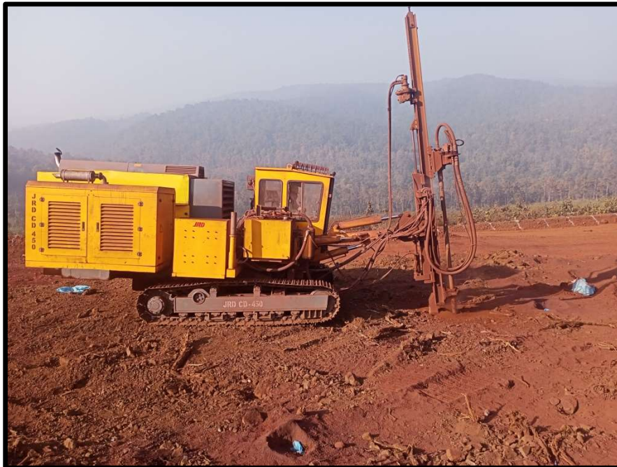
PHOTOGRAPH: 8 PHOTOGRAPH SHOWING VIEW OF WET DRILLING
