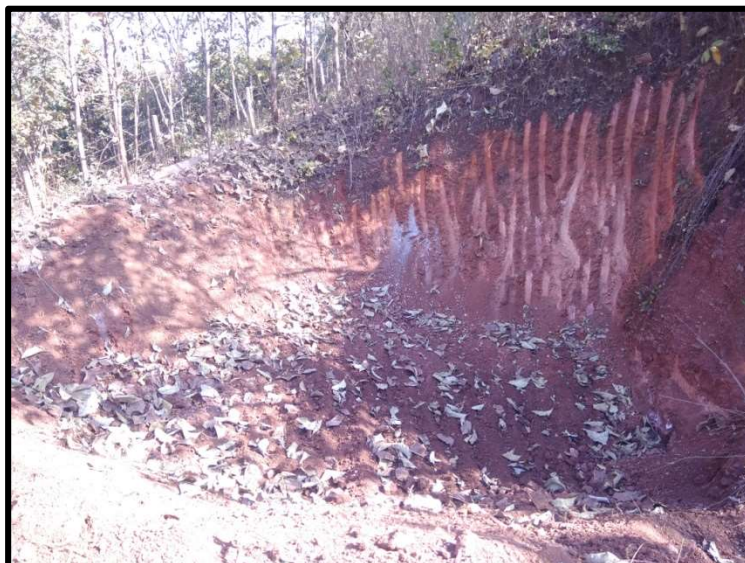
PHOTOGRAPH: 7 PHOTOGRAPH SHOWING VIEW OF RECHARGE POND
