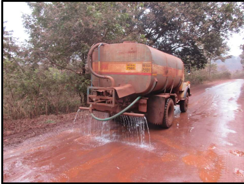
PHOTOGRAPH: 10 PHOTOGRAPH SHOWING VIEW OF WATER SPRINKING
