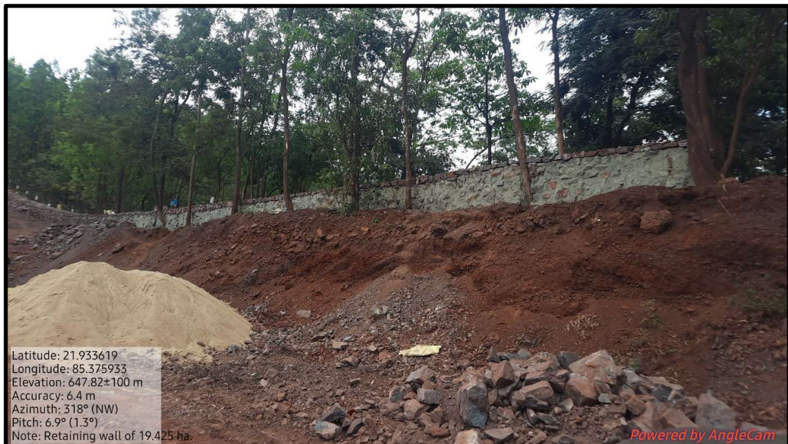
PHOTOGRAPH: 4 PHOTOGRAPH SHOWING VIEW OF CHECK DAM/RETAING WALL
