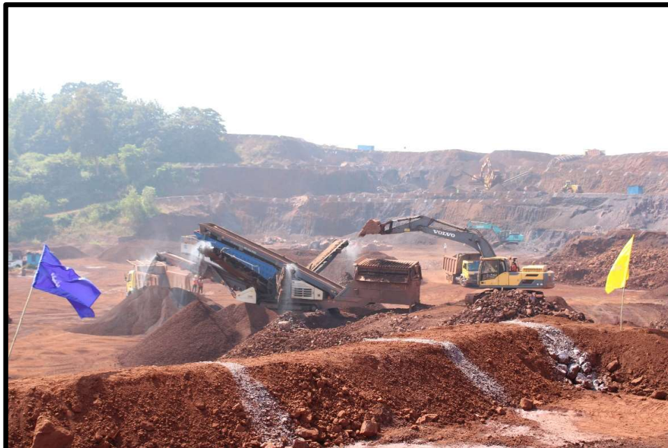
PHOTO: 14 PHOTOGRAPH SHOWING CRUSHING AND SCREEN PLANT IN OPERATION
