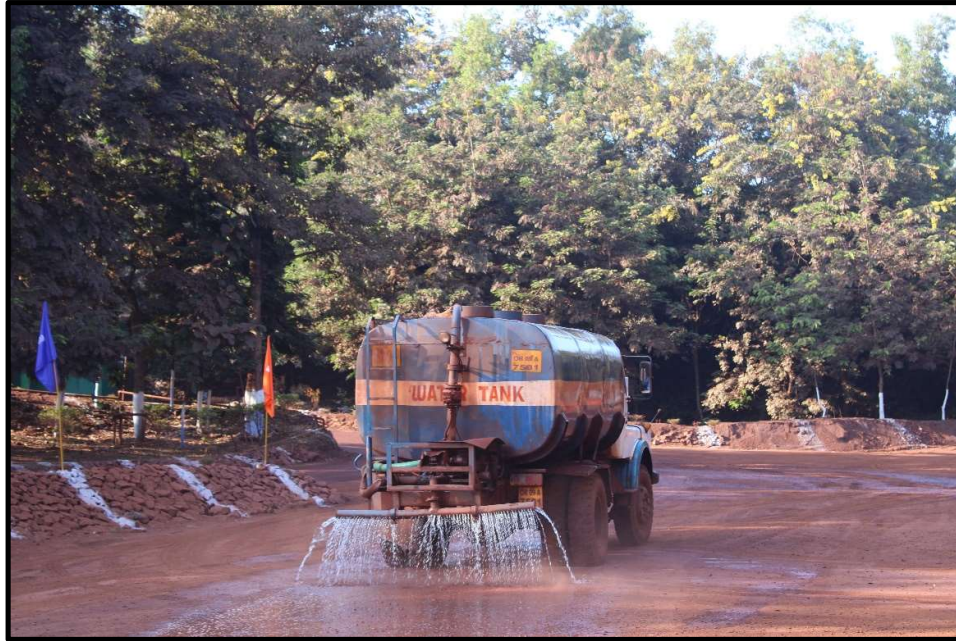
PHOTO: 11 PHOTOGRAPH SHOWING WATER SPRINKLING
