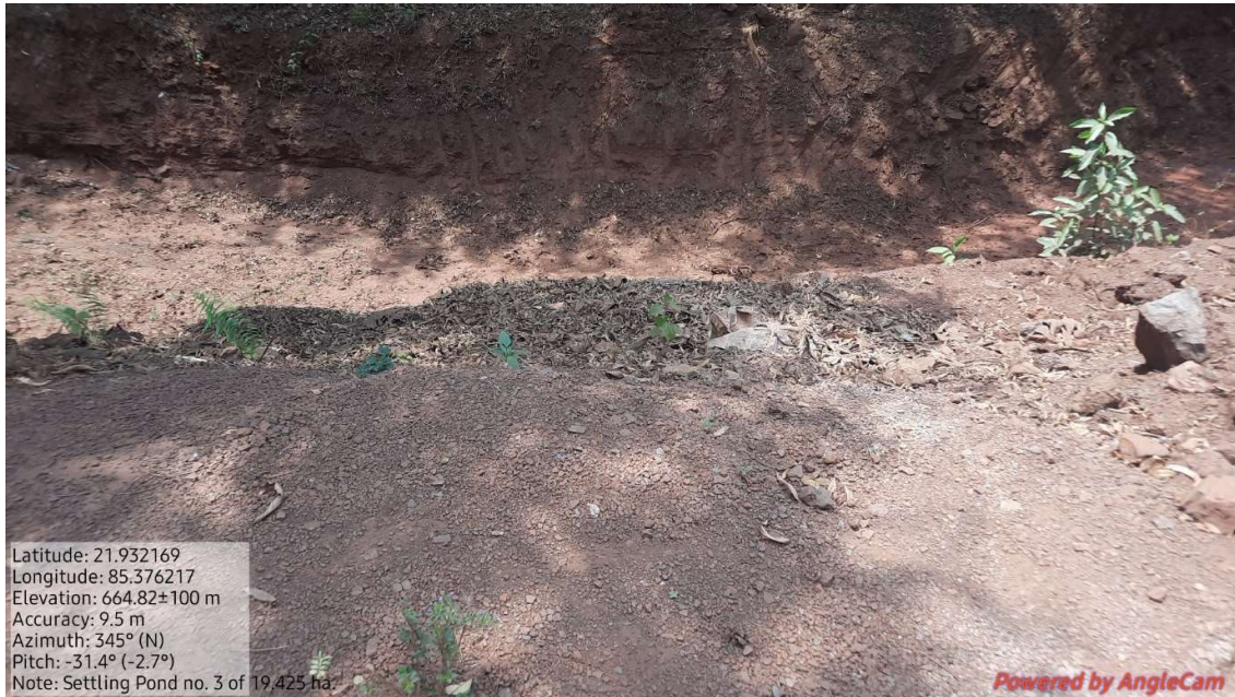
PHOTO: 13 PHOTOGRAPH SHOWING RAINWATER HARVESTING POND
