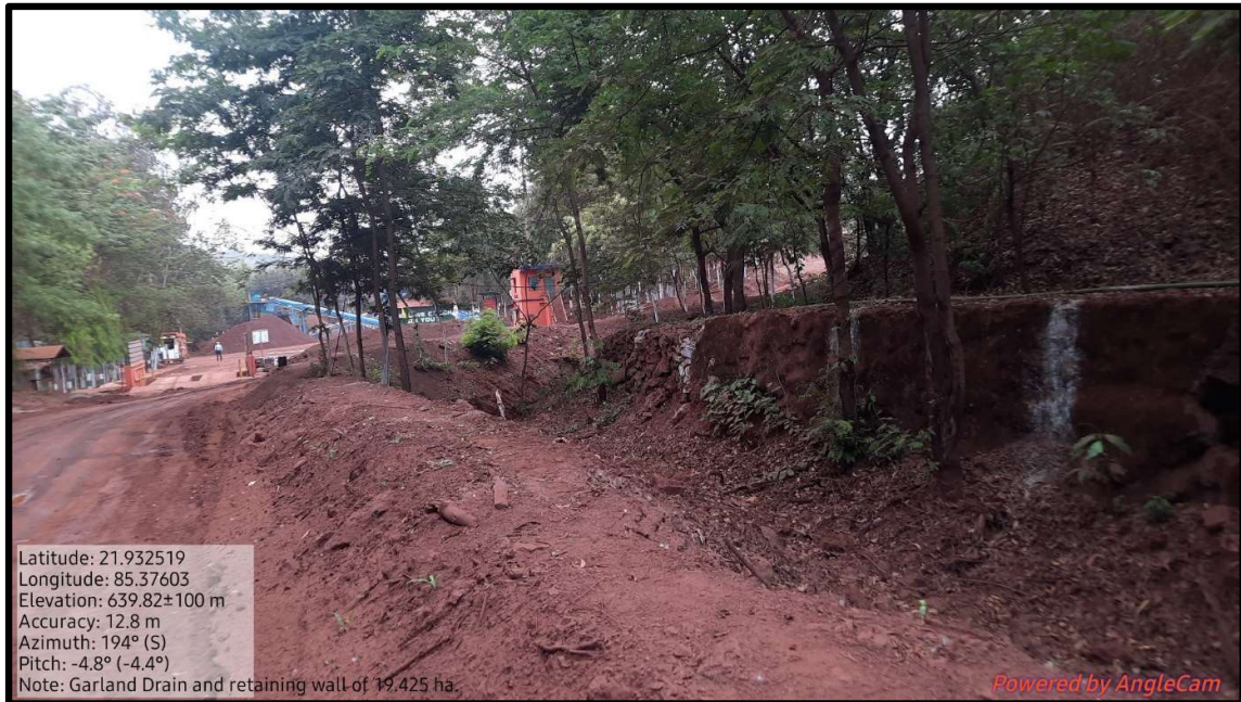
PHOTOGRAPH: 3 PHOTOGRAPH SHOWING VIEW OF GARLAND DRAIN AND RETAINING WALL
