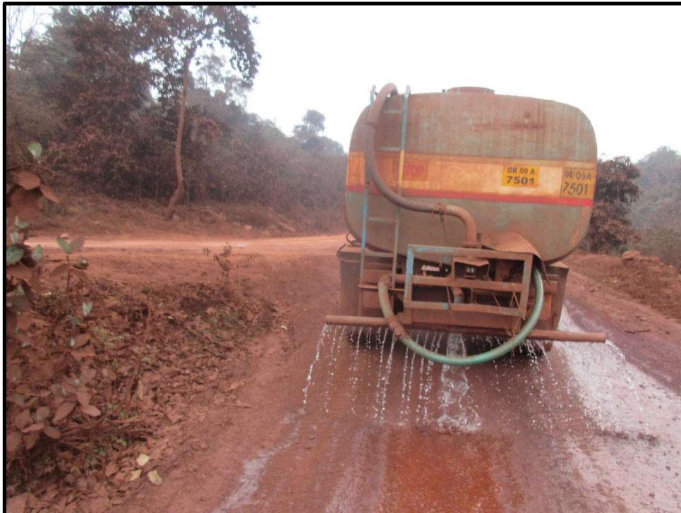
PHOTO: 12 PHOTOGRAPH SHOWING WATER SPRINKLING OUT SIDE ML AREA
