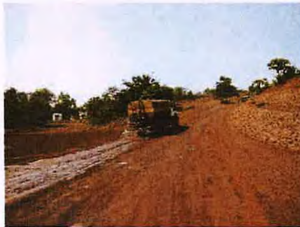
WATER SPRINKLING ON HAUL ROADS
