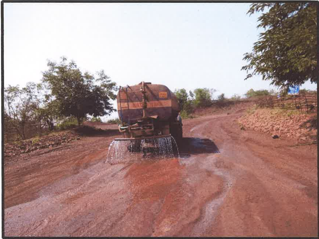
WATER SPRINKLING ON HAUL ROADS
