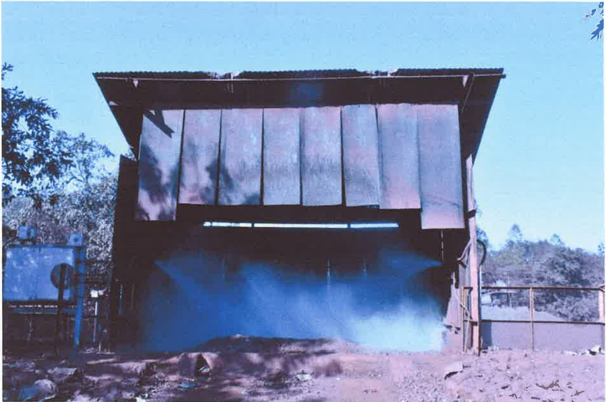
DRY FOG SYSTEM IN WORK
