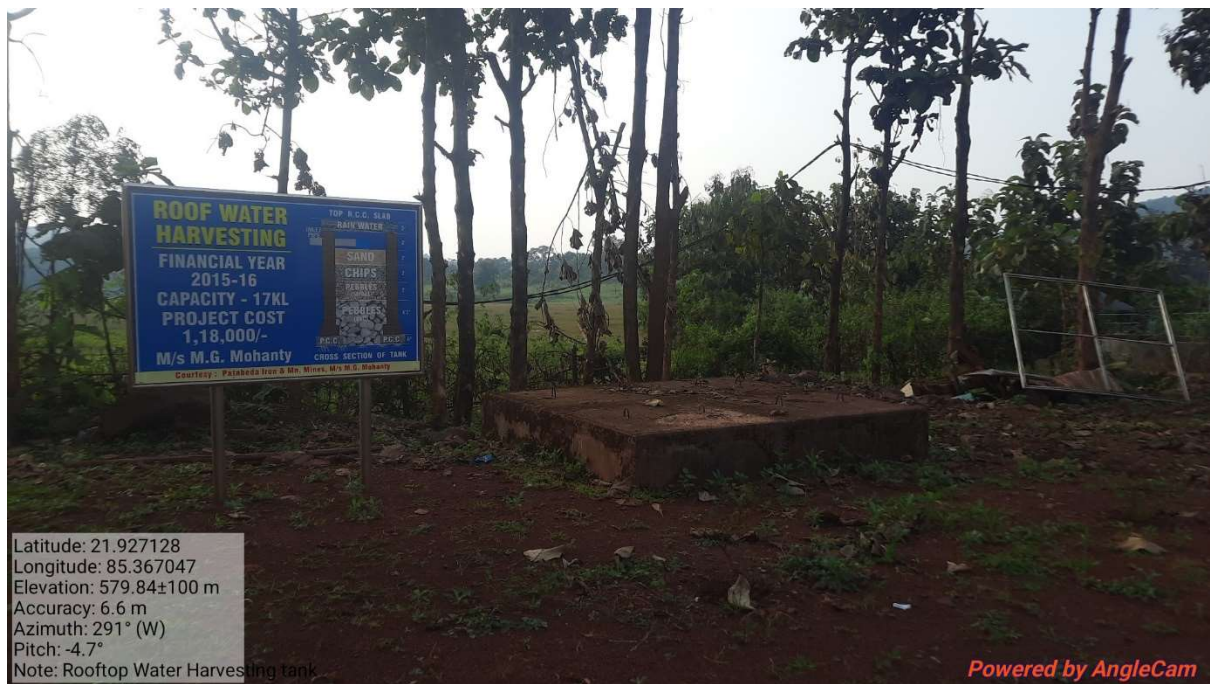
PGOTOGRAPH OF ROOF TOP WATER HARVESTING WELL
